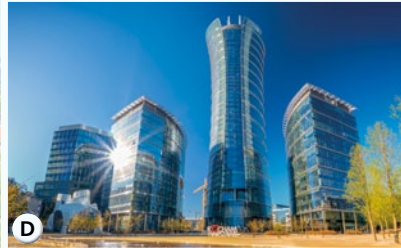
Warsaw Spire, Warsaw
