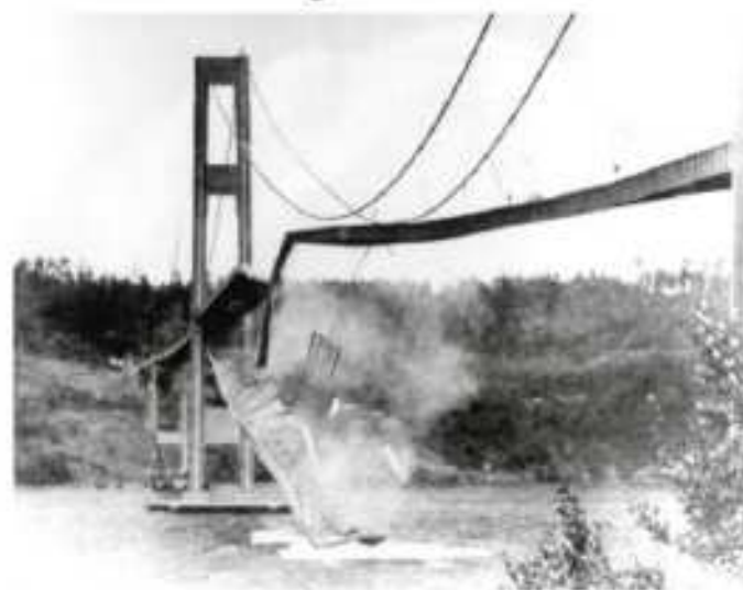
Rys. 25. Katastrofa mostu Tacoma Narrows.
